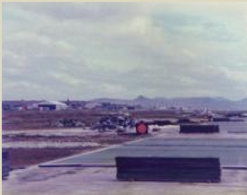
1986/87 Stanley Airfield Lifting M2 Matting Photo courtesy of 'arthurdaily' from the Sapper Site
