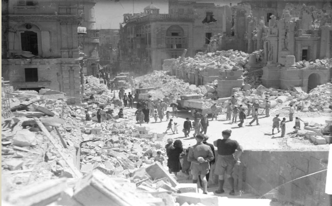
A heavily bomb-damaged street in Valletta, Malta. This street is Kingsway, the principle street in Valetta. Service personnel and civilians are present clearing up the debris.
